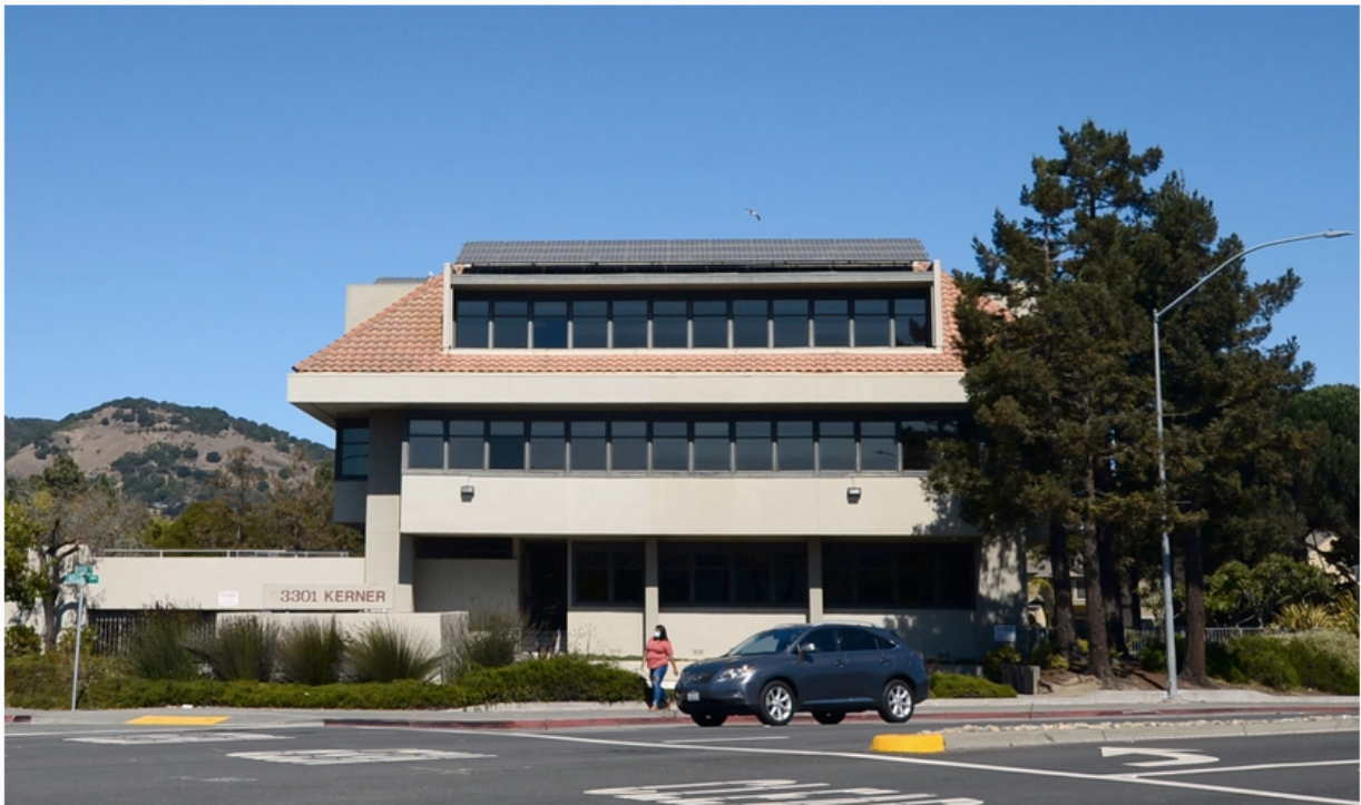
The vacant office building at 3301 Kerner Blvd. in San Rafael, Calif., on Wednesday, Sept. 23, 2020. Homeward Bound of Marin plans to use the top floor as a homeless shelter. (Sherry LaVars/Marin Independent Journal)
